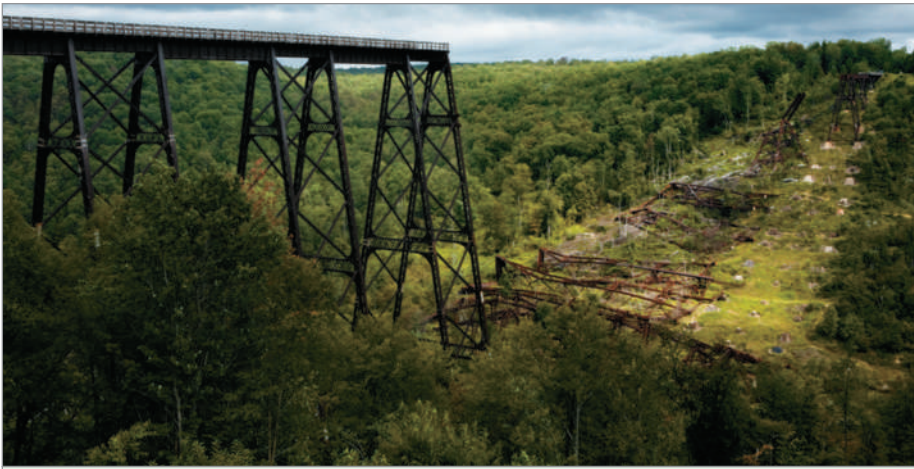
The Kinzua Viaduct Bridge in northwest Pennsylvania, constructed in 1882, was the longest railroad bridge in the world, spanning 2,053 feet and reaching a maximum height of 301 feet. It facilitated the flow of raw materials from the east to the great lakes regions. The trestle bridge was destroyed by a tornado in 2003. It takes reminders such as this to highlight the importance of integrated supply chains to avoid disrupting the flow of products and supplies.
