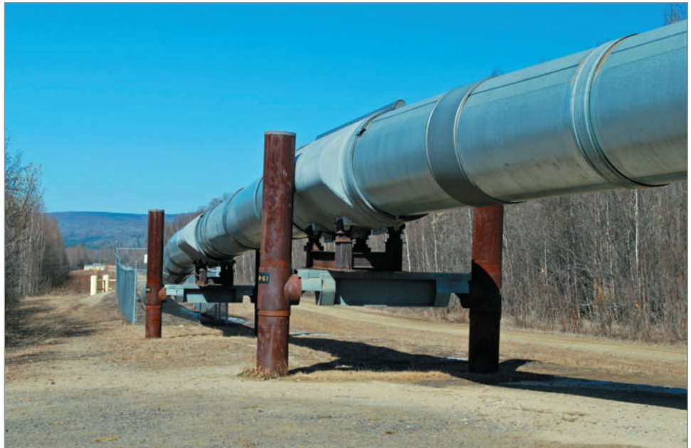
The Trans Alaska Pipeline System traverses 800 miles from the North Slope of Alaska to the northern most ice-free port of Valdez, Alaska. The pipeline is 48 inches in diameter, has 11 pump stations, and has a maximum throughput of 2 million barrels per day.
